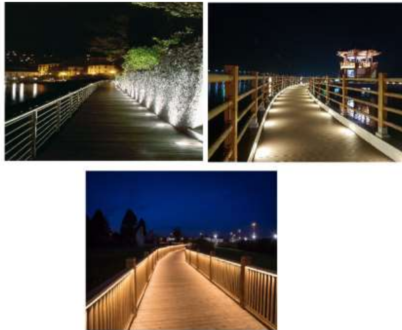
Gambar. Contoh Ilustrasi Panduan Lampu atau Penerangan Boardwalk up light lighting (kiri), recessed lighting (kanan) dan strip lighting (bawah).
