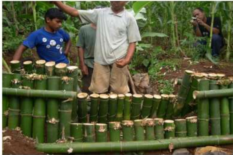
Gambar 4.45. Bio Gully Plug tampak depan di lapangan
